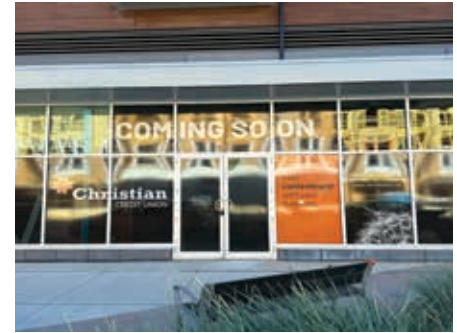
Construction progress as of Sept. 7, 2024.
